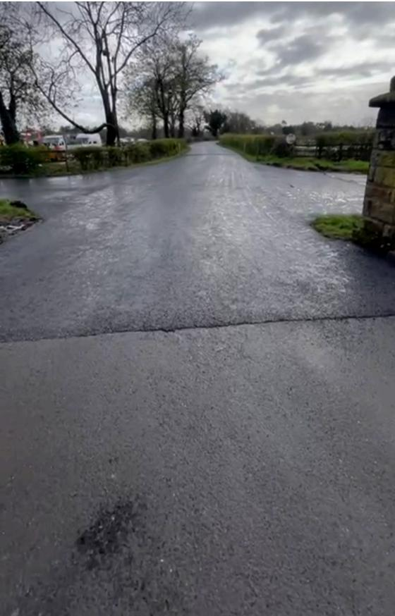
Our Work: An old concrete road over a mile long used by heavy traffic accessing a busy hotel and riding club is severely cracking and deteriorating.
